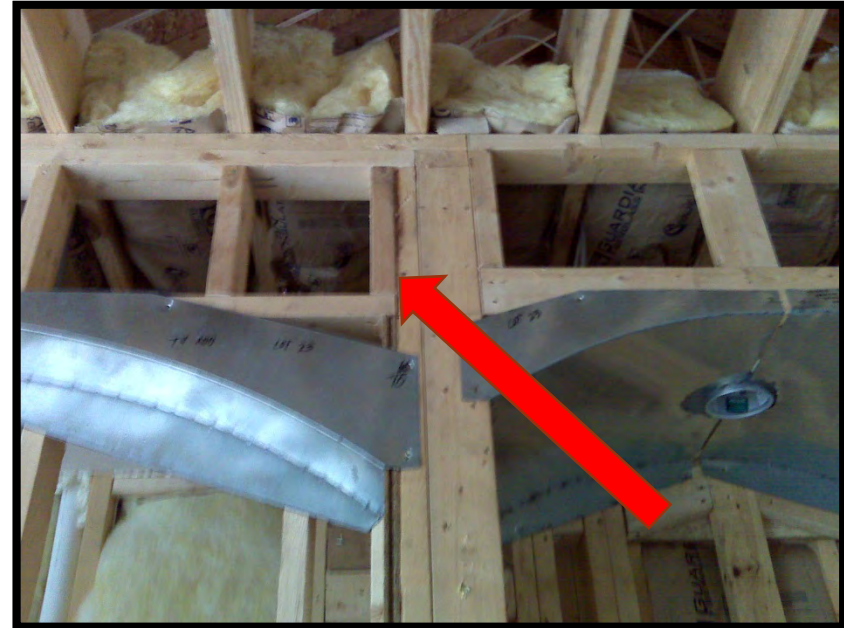
402.4.1 Building thermal envelope. - 3. Cap and seal soffit or dropped ceiling
