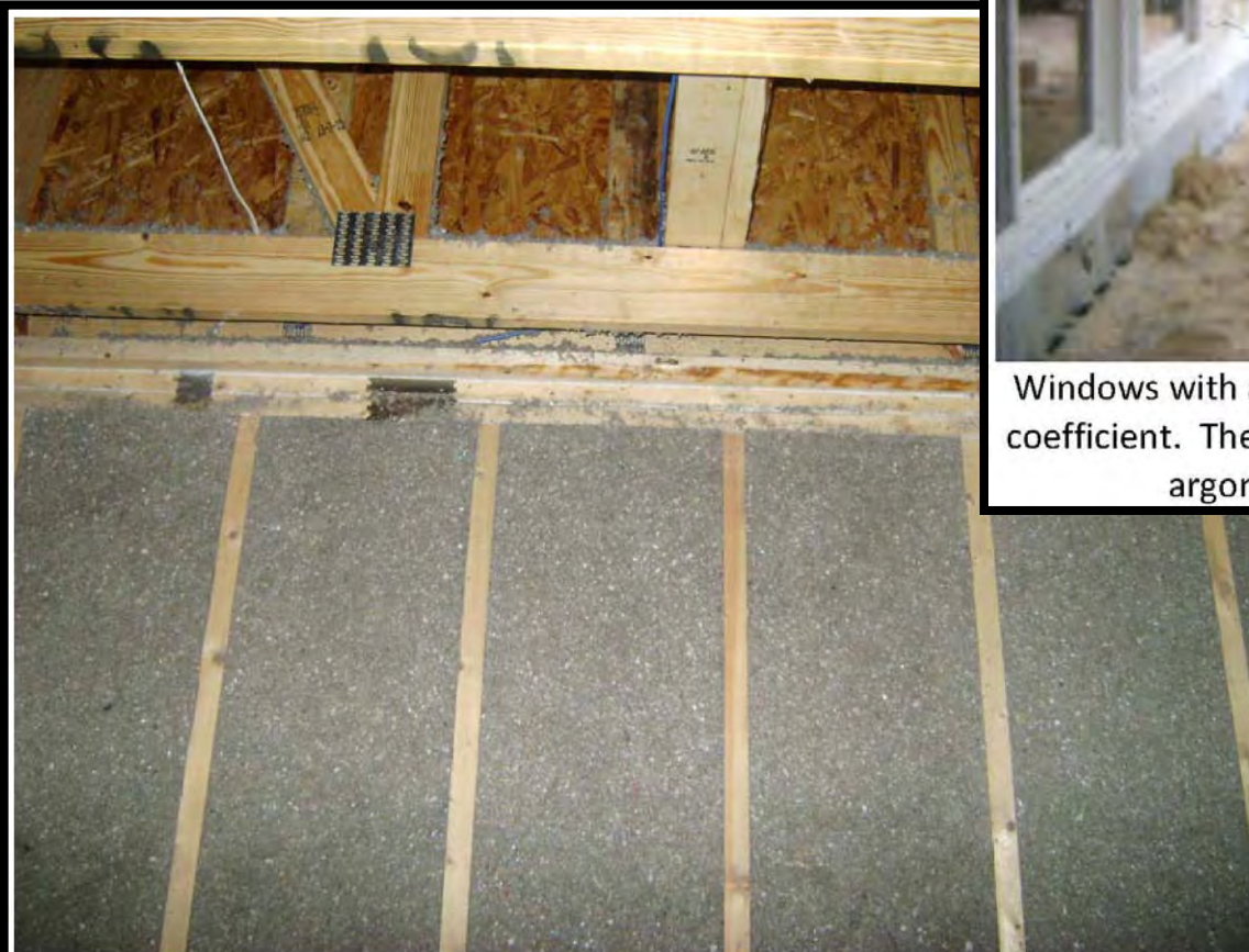
Grade 1 blown-in cellulose insulation. Double top-plates caulked to minimize air infiltration.
