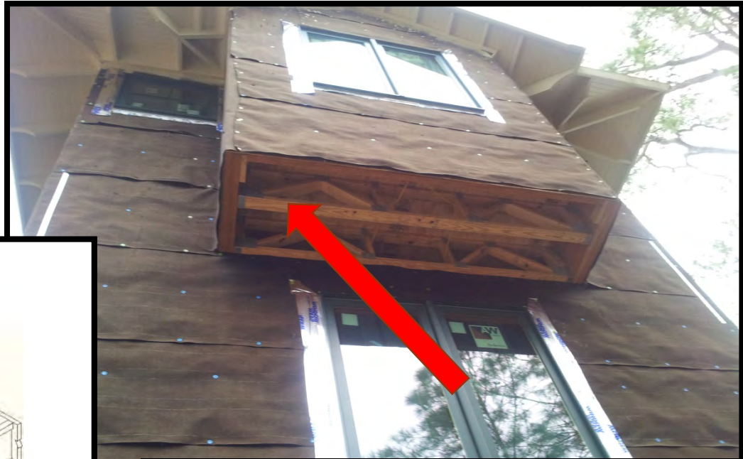
402.4.1 Building thermal envelope, – 1. Block and seal floor/ceiling systems
