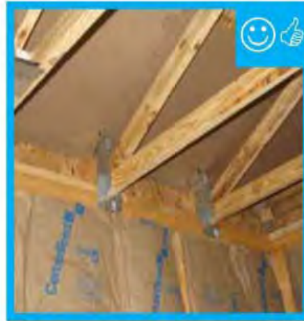
Wind baffle installation will allow proper insulation depth over the top plate.
