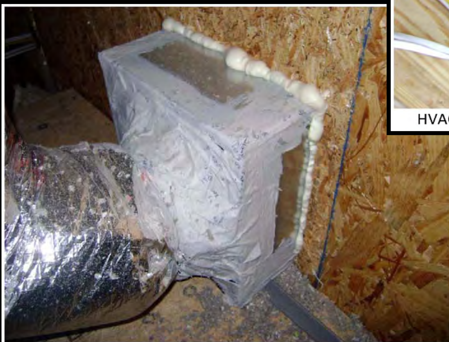
Return duct completely sealed using a paint on mastic product. Return boot sealed with foam at wall penetration.
