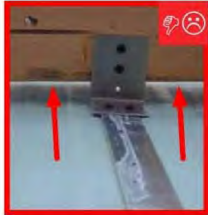
A. Air leakage path in a common wall.
