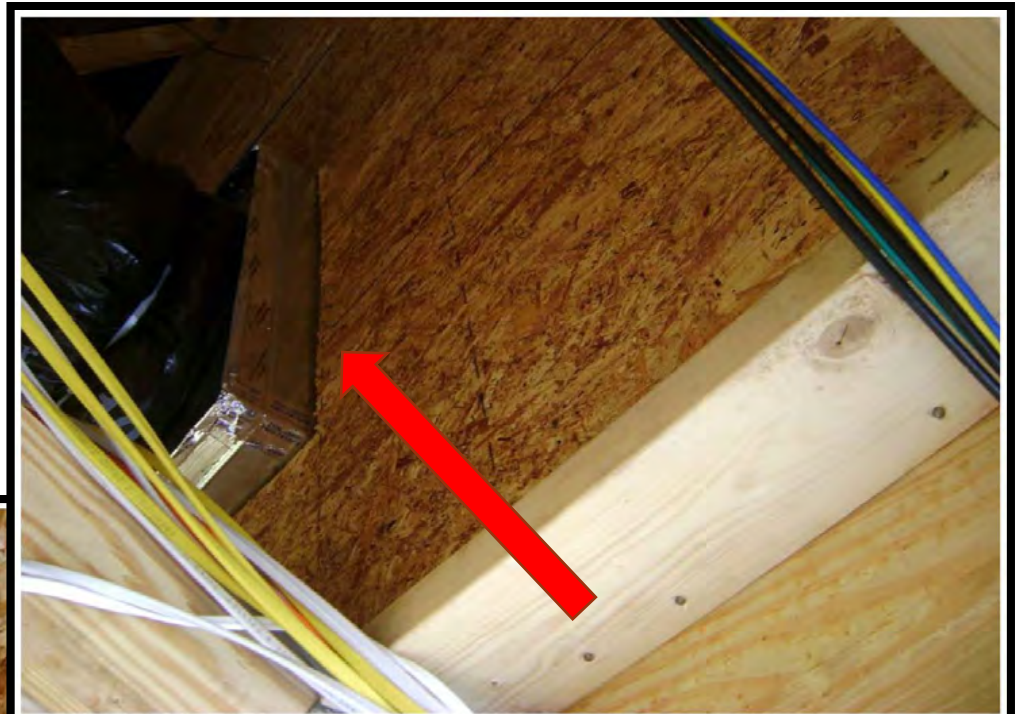
HVAC return should be caulked around knee-wall penetrations.
